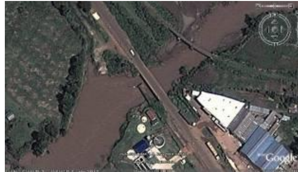
Nzoia River crossing at Mois Bridge
