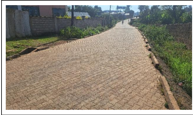
Plate 5-24: Section of the Hospital -Kiramburine Road paved with cabro
