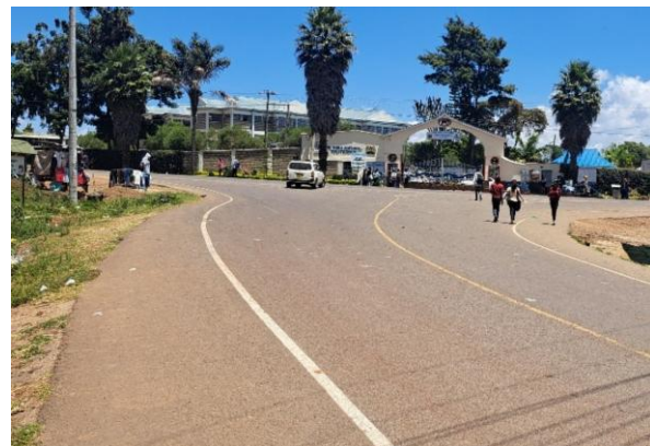
Plate 5-23: Tarmacked Western Bypass Road at the Meru National Polytechnic T-Junction
