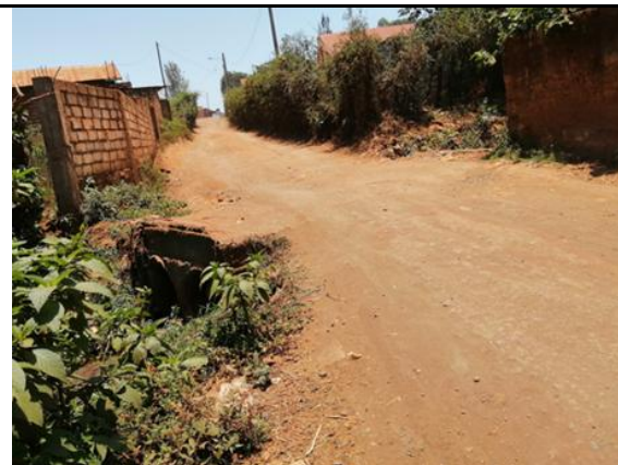
Plate 2-10: A cross culvert on Link 3-MeWASSCO Junction Road
