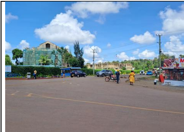
Plate 2-13: Photograph showing the location where the footbridge is proposed to be constructed
