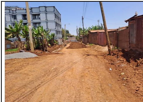
Plate 2-9: A section of Hospital Road Kiramburine JCT Road under construction
