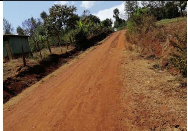
Plate 2-8: Road section at the end.
