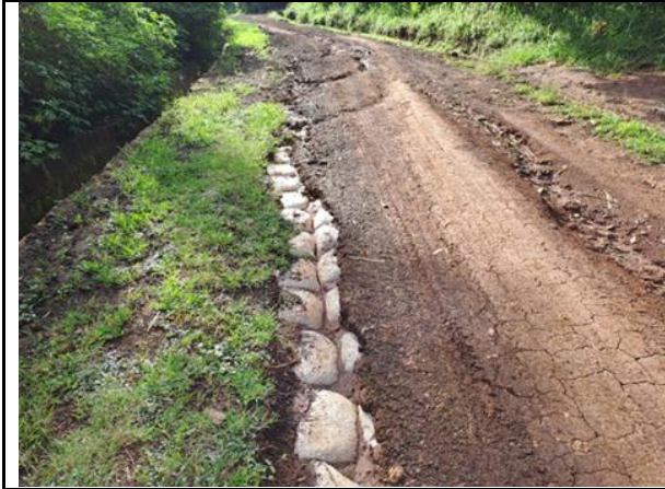
Plate 2-11: Exposed gunny bags filled with gravel
