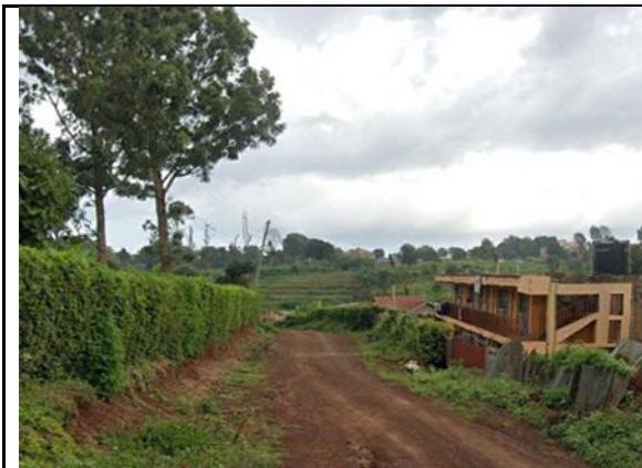
Plate 2-5: A gravel section of the Road
