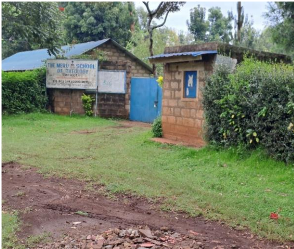
Plate 5-18: Meru School of Theology at Km 0+600 RHS of the Kambakia-Kagotone Road (Apprx 150 meters)
