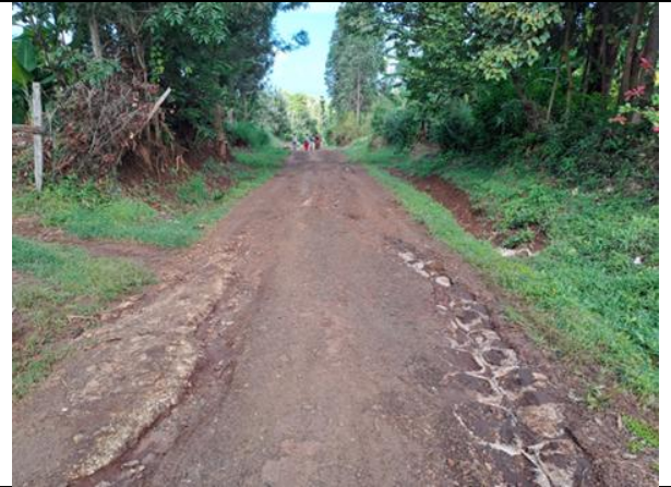
Plate 2-12: Gunny bags filled with gravel showing signs of erosion.
