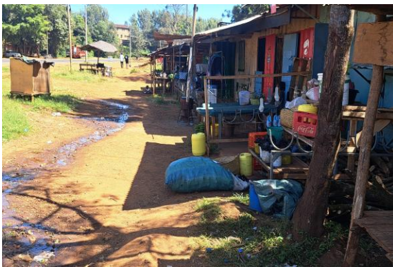
Plate 5-14: Business sheds at the end of Kambakia - Kagotone/KEMU Road
