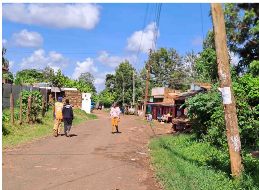
Plate 10-3: Some of the Business at Km 0+150 Western Bypass Link - Mate Road
