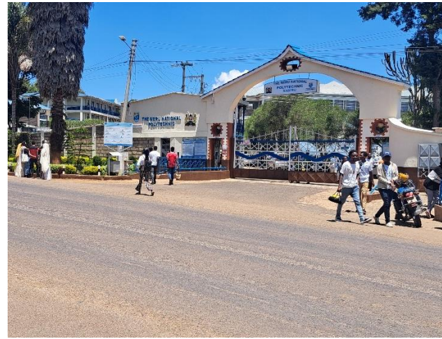
Plate 5-19: Meru National Polytechnic along the Meru Nanyuki Highway
